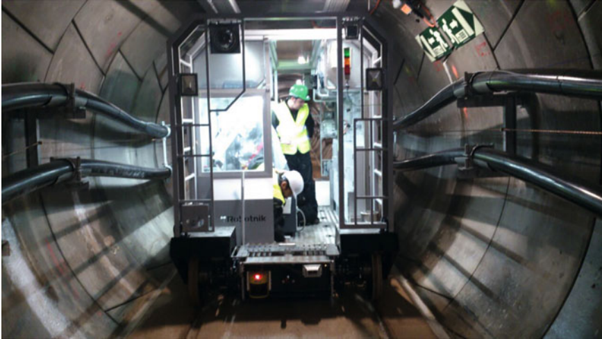
Fig. 6 R-INSPECT Autonomous Inspection Robot inside the tunnel
