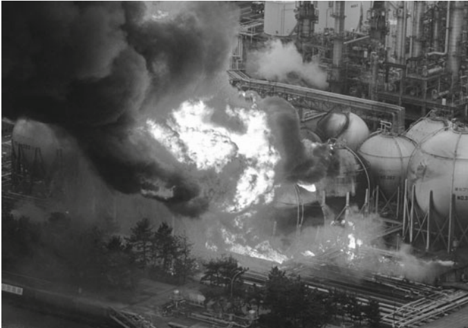
Fig. 1 Major failure and explosion of a LPG tank
