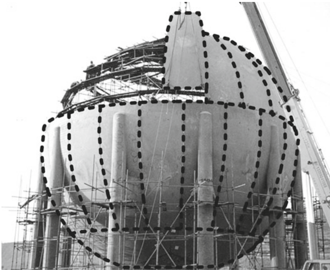
Fig. 6 Assembly of a LPG Sphere tank with digitally highlighted weld beads
