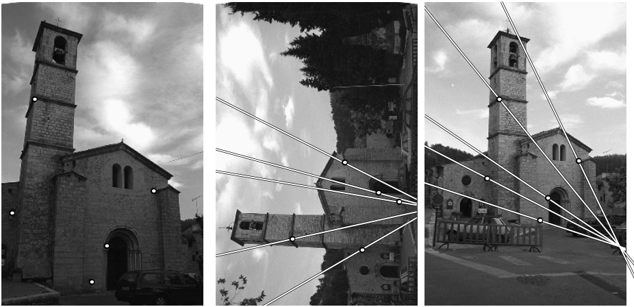
Fig. 6. Wide baseline matching. Three images acquired from very different view-points with a hand-held camera. The trifocal tensor is estimated automatically from interest point matches and a global homography affinity score. Five of the matched points are shown together with their corresponding epipolar lines in the second and third images. The epipolar geometry is determined from the estimated trifocal tensor. Original images courtesy of RobotVis INRIA Sophia Antipolis. The wide baseline method is described in [25].
